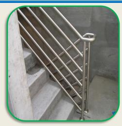
STAINLESS STEEL HANDRAIL WITH NO MIDDLE BALUSTRADS
