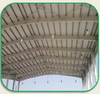
Steel structure with sandwich panel
